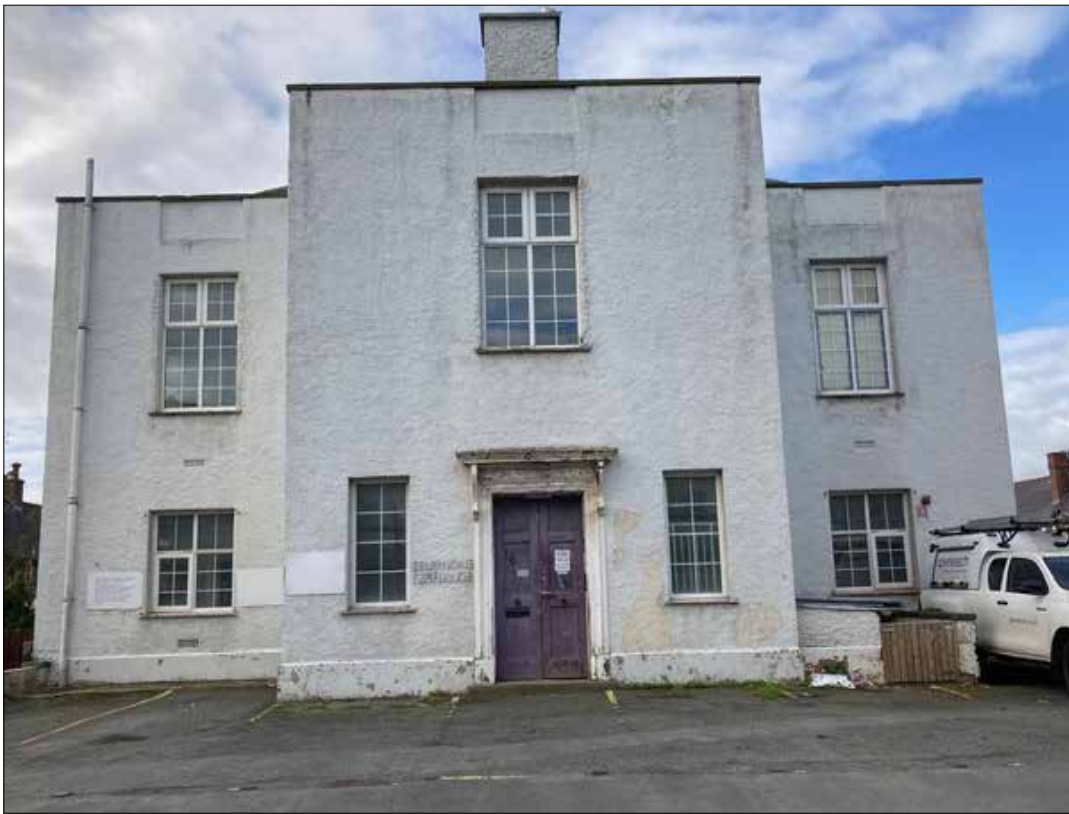
Albert Road Telephone Exchange.
