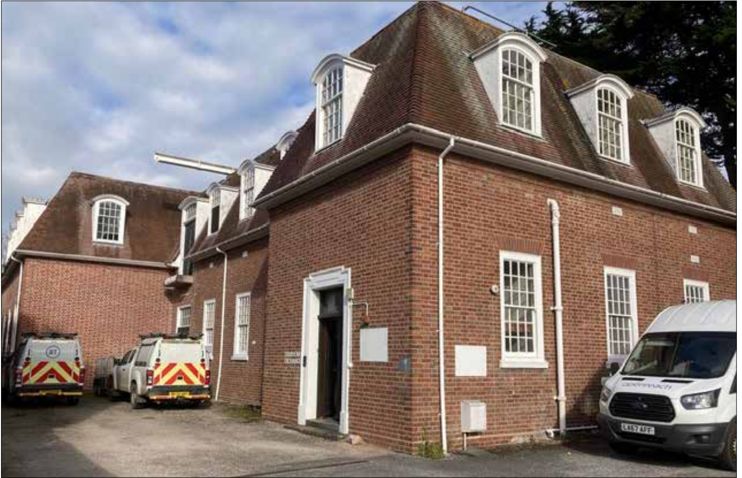
Allanson Road Telephone Exchange.
