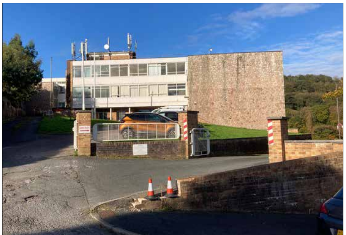
Conwy Road Telephone Exchange.
