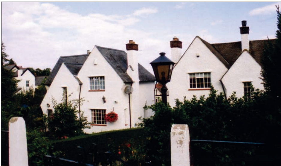
Number 6 (left) and 4 (right) Ael-y-Bryn Road. No 6 was his own. No 4 built for Ken Neill
